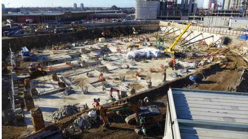
Figure 3: Preparation of the mat slab foundation, February 2014. (Department)
