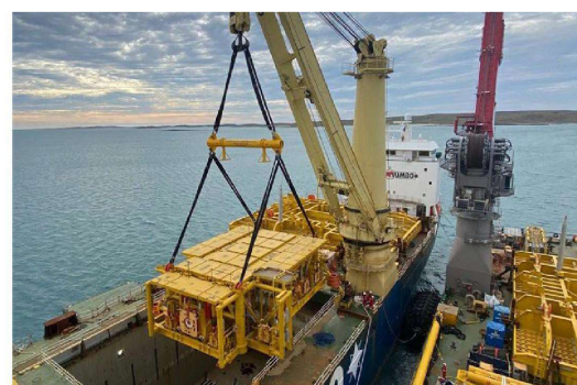
Gorgon Stage 2 Manifold Lift (370 tonnes)
