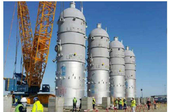
Tengiz Area 42 sieve vessels Train 2 foundations
